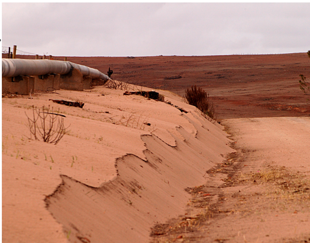
Soil erosion after a bushfire.
